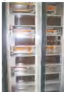
Internal separation form 4
