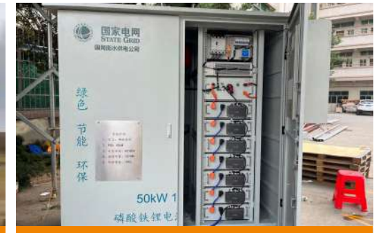
China State Grid 50kW/100kWh energy storage system
